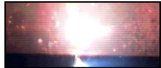
High Level Arcing (>100 Amps) After Flashover
